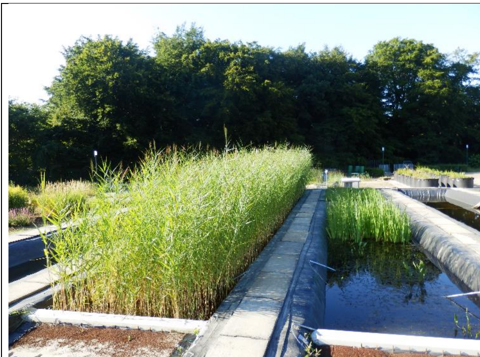
Figure 1: The pilot treatment systems at the Radboud University in Nijmegen. On the left the traditional reed-filter, and on the right the biocascade with (from the front to the back: iron coated sand filter, Myriophyllum compartment and the Iris compartment.
